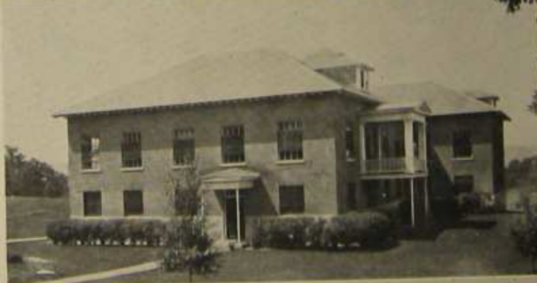
TOP TO BOTTOM— DORMITORIES "A" "C", "D" AND "E"
